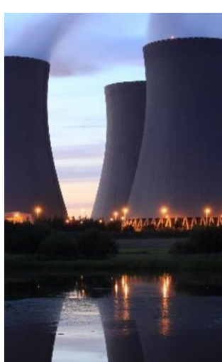
Critical Infrastructure & Industry
