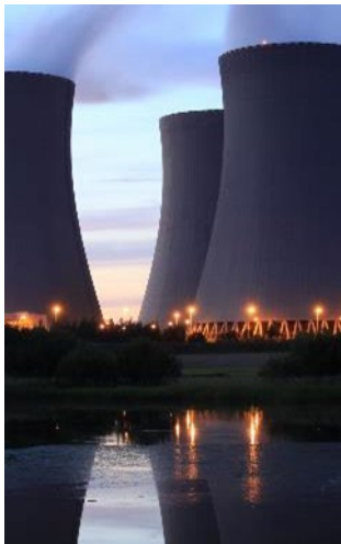
Critical Infrastructure & Industry
